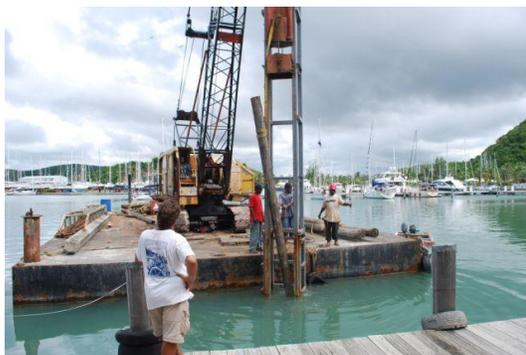
**JOLLY HARBOUR** - permission has been given by the development company C.D.A.L. and Mr Charles Kenlock of Jolly Harbour Marina for us to create the necessary infrastructure. The piles have been driven to support the launch ramp for the dinghies and the boats will be housed in a fenced compound provided by C.D.A.L. We have still to construct the launch ramp and plans for this are in hand.
