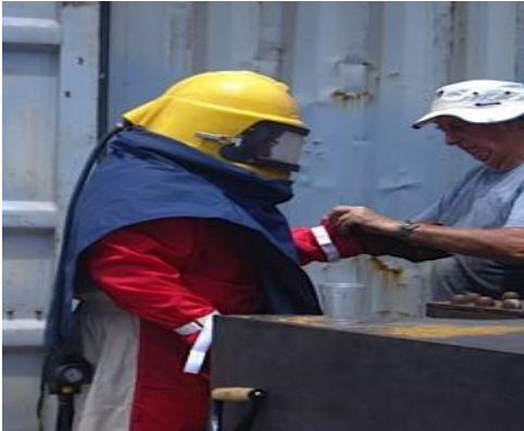
Serious sand blasting equipment. Lawrence Gameson suited up.
