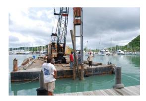
JOLLY HARBOUR - permission has been given by the development company C.D.A.L. and Mr Charles Kenlock of Jolly Harbour Marina for us to create the necessary infrastructure. The piles have been driven to support the launch ramp for the dinghies and the boats will be housed in a fenced compound provided by C.D.A.L. We have still to construct the launch ramp and plans for this are in hand
