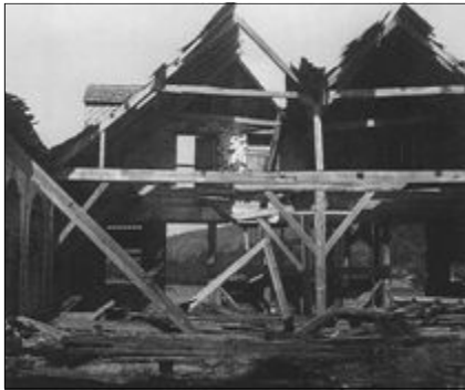
In 1948, prior to renovation, this was all that remained of the Cordage and Canvas store (Photos taken from 'Antigua and Barbuda Photographic Journey' )
