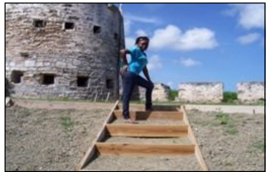
Teacher Jarvis strikes a pose at the historical Martello Tower which is presently under renovation.
